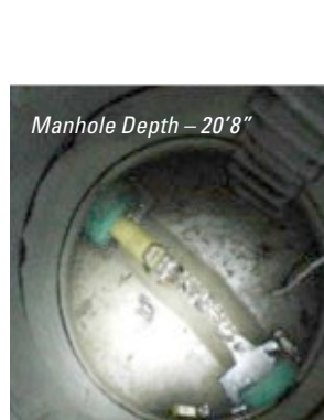
Figure 1: Photo of manhole
